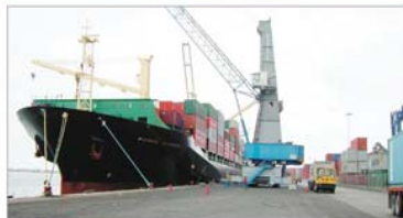
The Ecuadorian container terminal, Puerto Cabello, the sixth largest port in South America is still lacking a quay crane.
